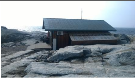
Utö measuring cabin outside
