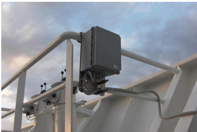
Telemetry box installed on bow open deck.
