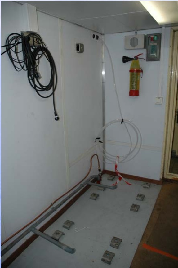
The lab has been prepared for installation of the AUMS (January 2011).
