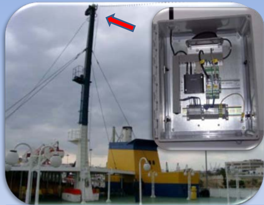
Positioning : GARMIN "Mouse" GPS-35 Communication: GSM Modem Siemens MC35. Installed on ships mast.
