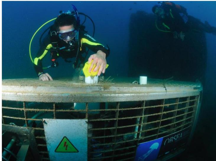
**Figure 13c.** *The cleaning of the underwater camera dome by divers at OBSEA.*
