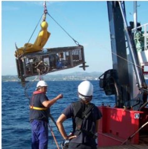
**Figure 4.** *On-board repair of the OBSEA submarine cable damaged during a maintenance operation of the junction box.*
