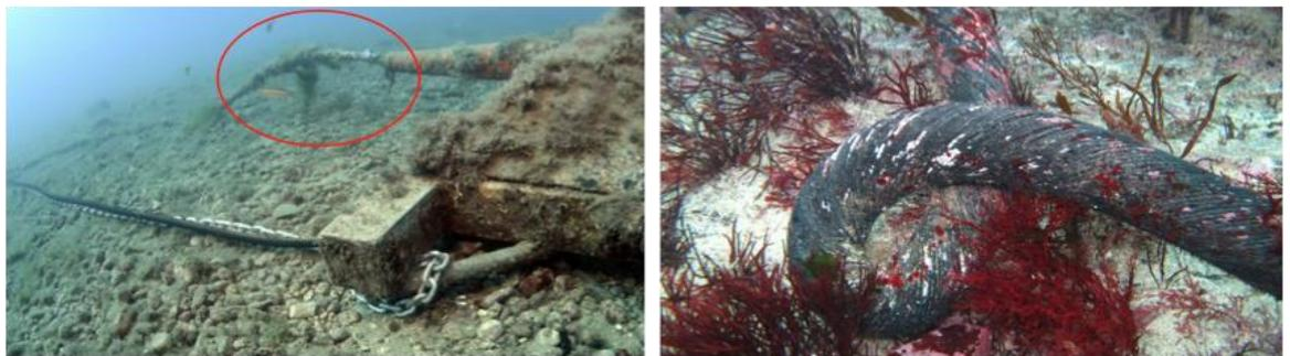
**Figure 2.** Common cable laying problems: too much or too little tension and friction can generate twists in a cable; cable overlap must be avoided at all costs.
