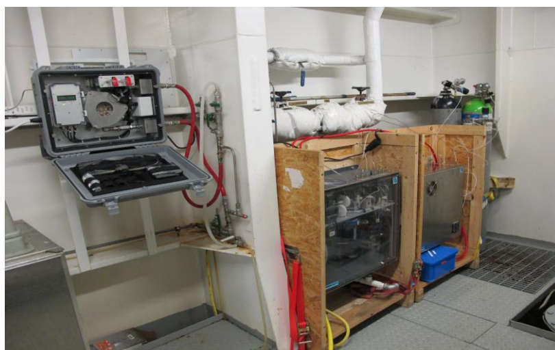
Figure 4.4.1. Installation of a NIVA-Franatech membrane based p\text{CO}_2 system (left) and a General Oceanic p\text{CO}_2 system (right). Test installation on the FerryBox system on MS Color Fantasy.
