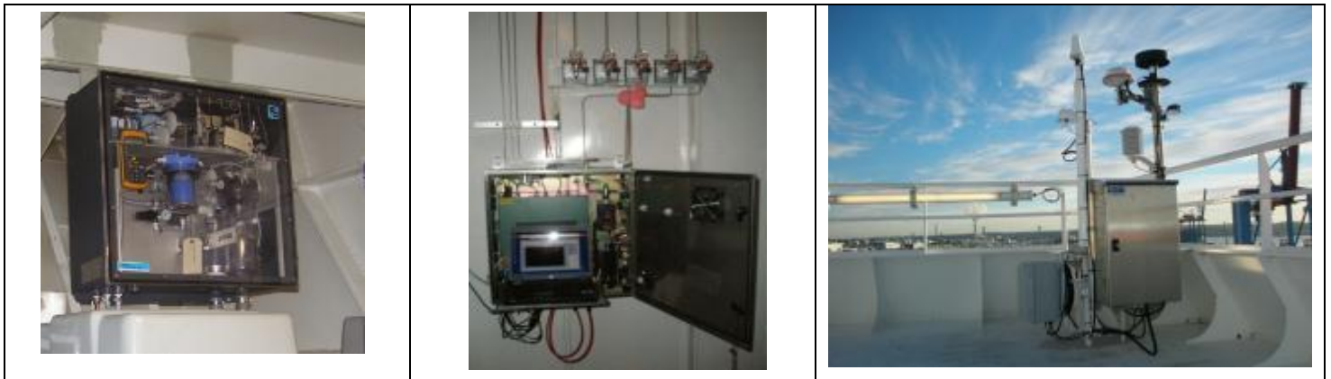
Figure 4.4.2. The General Oceanics 8050 \text{CO}_2 -system includes a wet unit (left) and a dry unit (middle) and a deck unit as well (right). The installation shown is on the ship TransPaper operating in the Baltic by SMHI.
