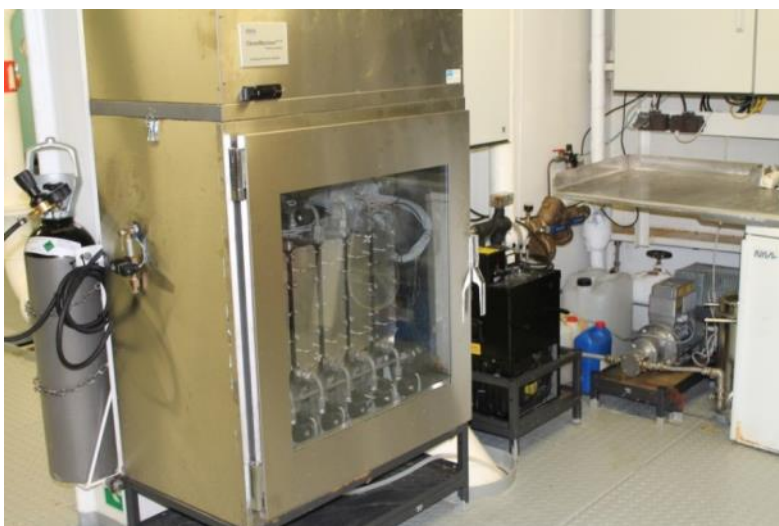
Figure 28 : Chem Mariner installed at MS Color Fantasy (left) and one of the chamber opened to illustrate the membranes (right). By courtesy of NIVA.
