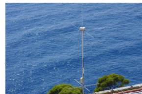
Compact transmitting and 3-element receiving antenna
